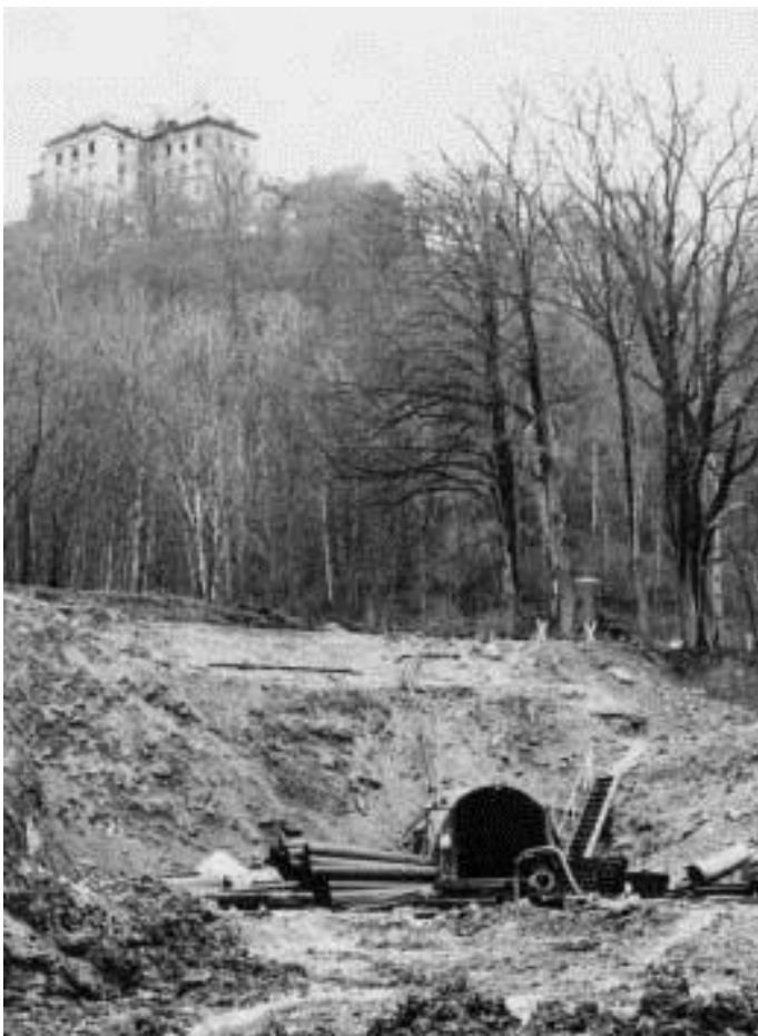
Survey gallery under Chateau Jezeří: main site of the detailed engineering geological survey
