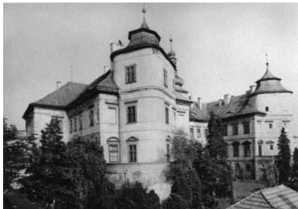
The right wing of the chateau rests on solid granite gneiss; the left wing stands on a fault zone, in which the rock is disintegrated into a sandy-clayey earth.
