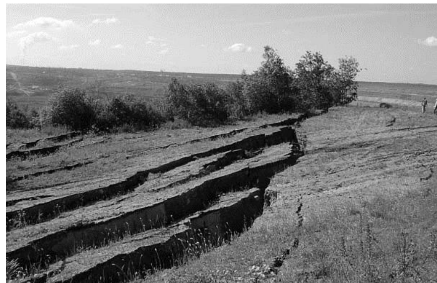
The large-scale open cast is a permanent threat to areas beyond the mining limits, as attested by the slide of about 3 million m 3 of earth in the arboretum protective column in June 2005.
